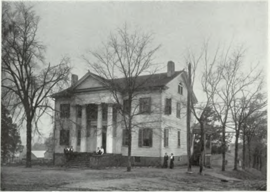
Newell House, Rented for Dormitory
