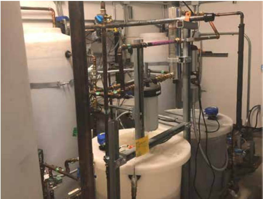
Figure 10. In house gray water recycling of the Architectural Nexus Salt Lake City Headquarters
