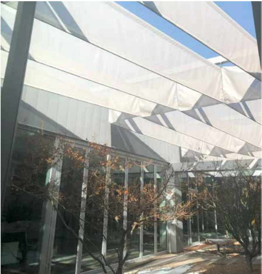
Figure 7. Atrium of the Architectural Nexus Salt Lake City Headquarters displaying ergonomic flap design
