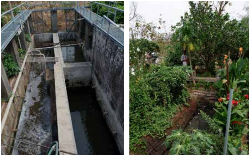
Figure 8. Two level gray water recycling system at Govardhan Ecovillage, India
