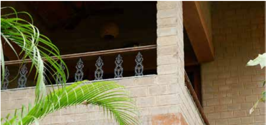
Figure 11. (Top) Compressed Stabilized Earth Blocks (CSEB) in Govardhan Ecovillage, India (Bottom) Community center at the Govardhan Ecovillage built using CSEB.
