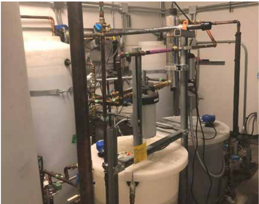
Figure 6. In house gray water recycling of the Architectural Nexus Salt Lake City Headquarters
