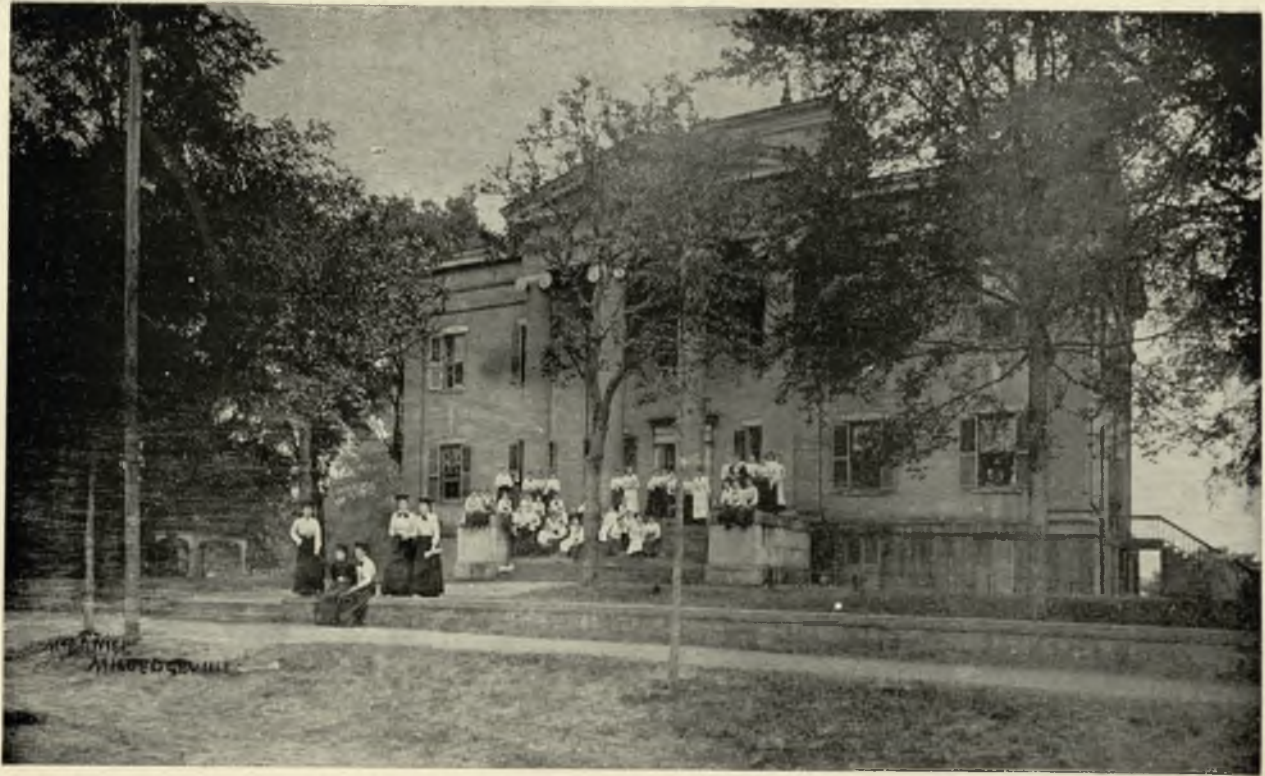
THE MANSION. (Part of Dormitory of the Georgia Normal and Industrial College.)
