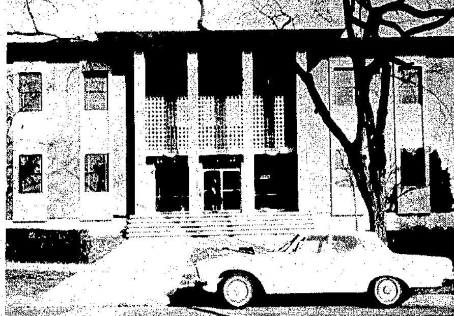
The new Home Economics Building
